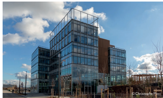
GA Smart Building
